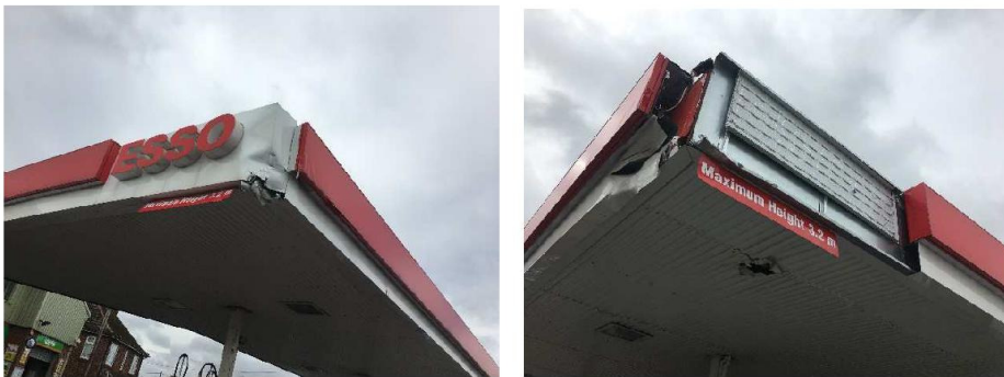
Figure 5 – Damaged Canopy
